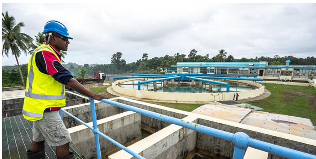
Existing wastewater treatment plants can co-treat fecal sludge with sewage if they can handle the additional load from septage and have facilities to separate liquids and solids. Photo credit: ADB.
