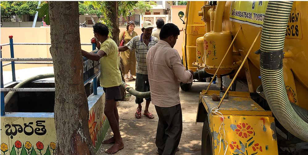
Emptying a vacuum tanker at a sewer discharge point in Visakhapatnam, India. Photo credit: Water & Sanitation for the Urban Poor.
