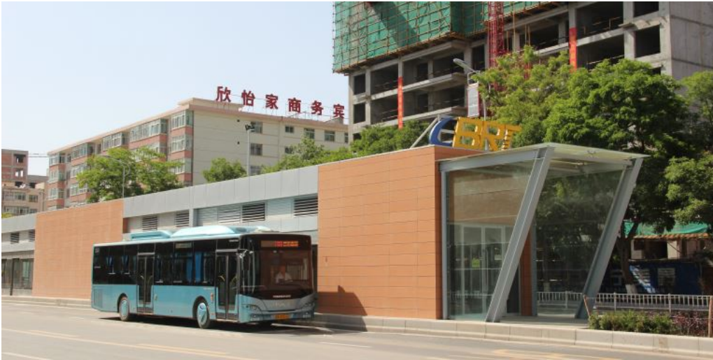
Lanzhou's Bus Rapid Transit as the centerpiece of its sustainable urban transport system
