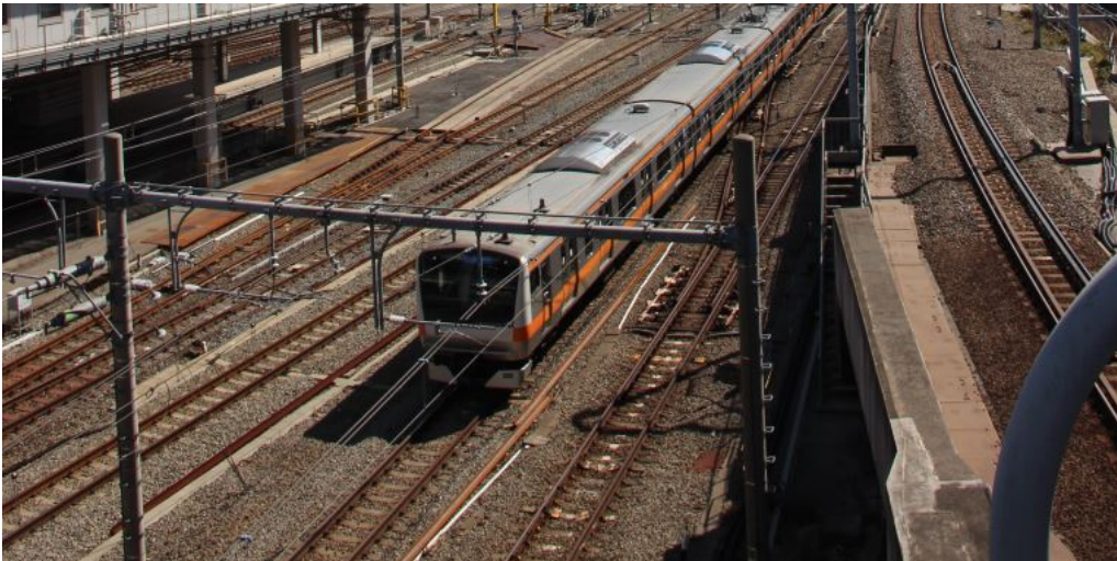
Shinjuku station in Tokyo, Japan is one of the busiest stations in the world in terms of passenger numbers, and is one of the successful models of transit-oriented development.
