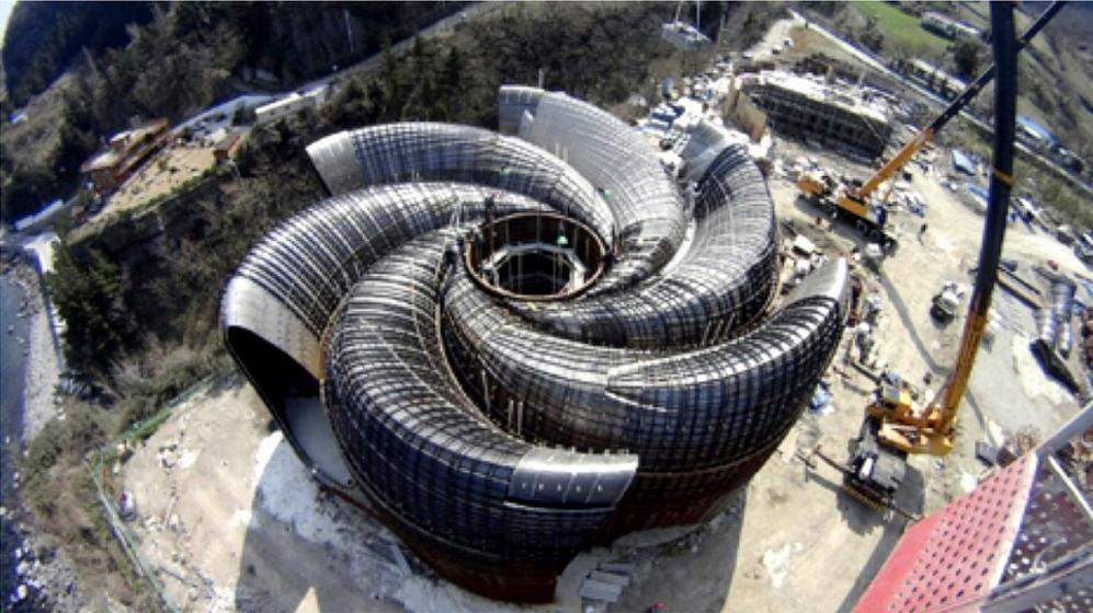
This is the formwork installation for SUPER Concrete pouring for KOSMOS – the world's first UHPC building structure. Photo credit: KICT, KOLON Global Co., The System Lab.
