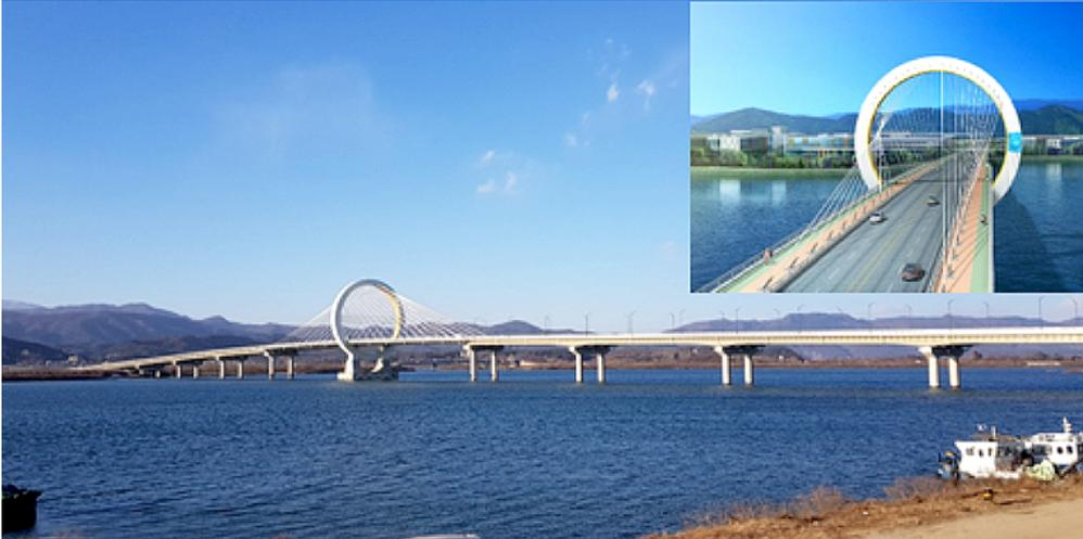
Chuncheon Grand Bridge, an access bridge to LEGOLAND Theme Park, is the first ultra-high performance concrete cable-stayed bridge in the world and was constructed using SUPER Concrete. Photo credit: KICT, Daelim Industrial Co.
