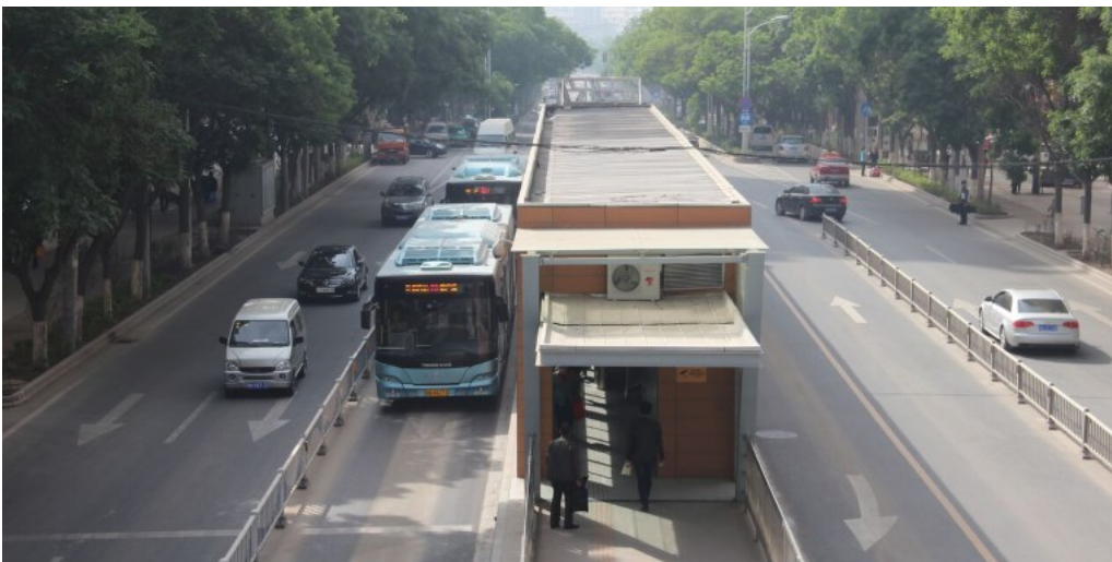
A key feature of the Lanzhou BRT is the split station design that allows buses going in the same direction to stop on either side of the station platform. Photo credit: Lloyd Wright/ADB.
