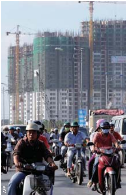
BUILDING BOOM Motorists ride past residential buildings under construction in Ho Chi Minh City, Viet Nam.
